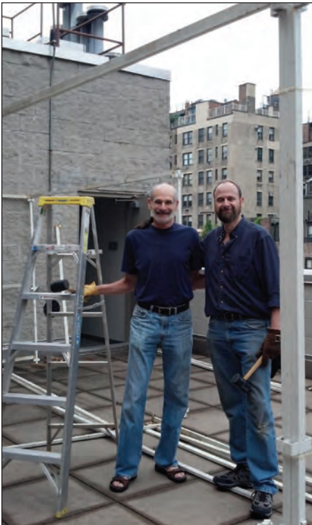
Building the sukkah.
